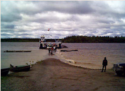
Ferry landing under high water.
