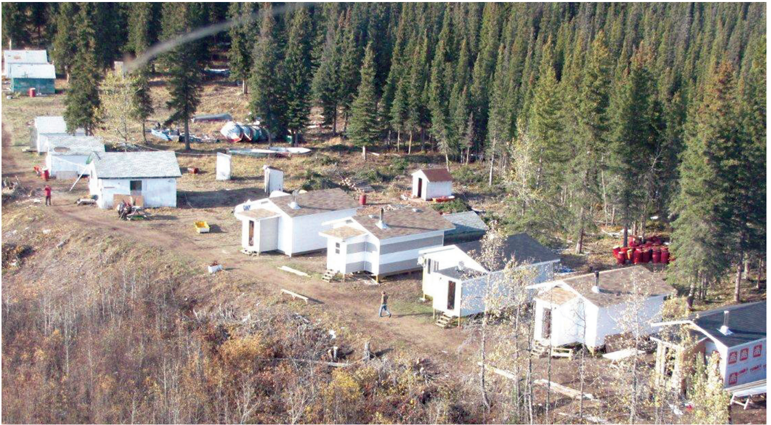
New cabins at Ten Shilling Creek, 2009.
