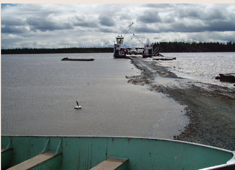
Ferry landing under high water.
