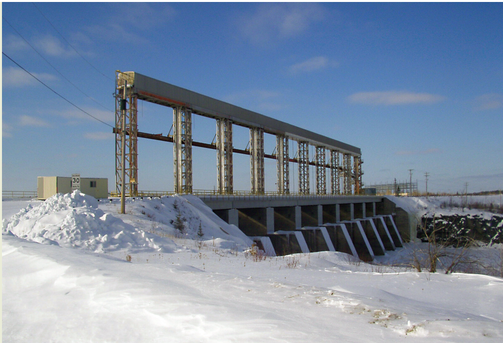
Kelsey Generating Station.
