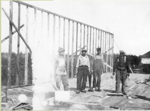
Building the Church at York Factory, 1933.
